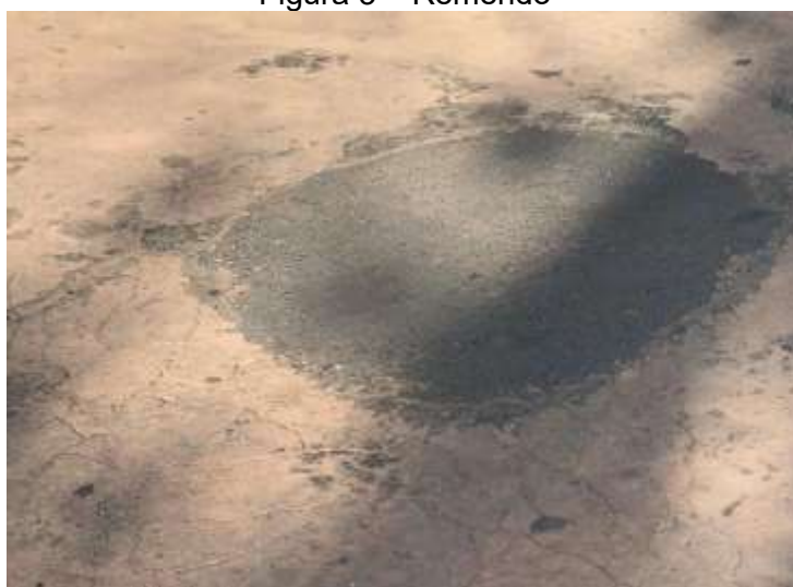
Figura 3 – Remendo
