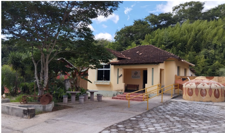
Main façade of the Living Center in Education Rural Sanitation in Florestal Source: courtesy photo
