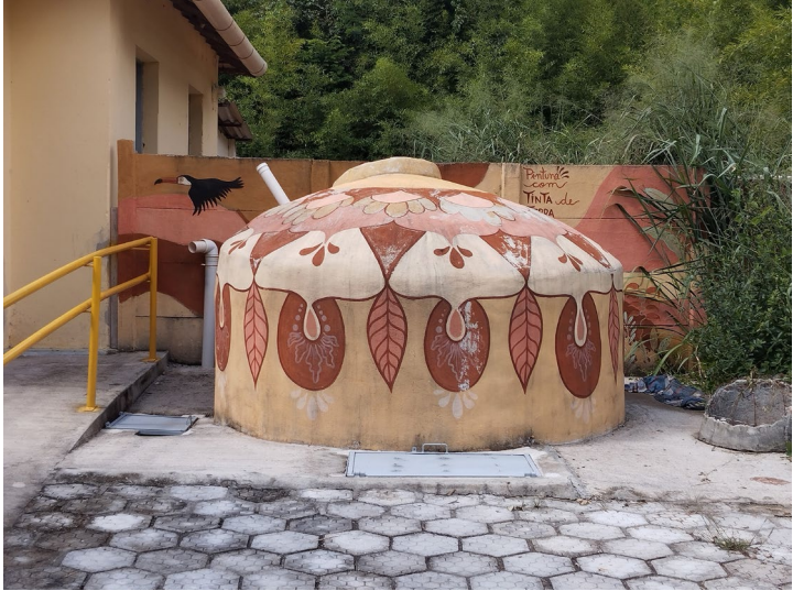
Rainwater collection cistern painted with natural dyes Source: courtesy photo
