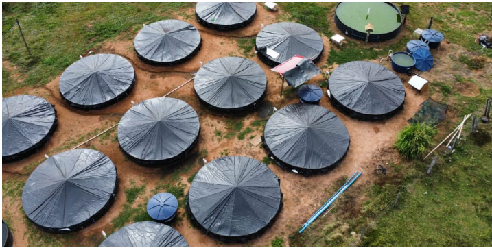
Tanks installed in a rural settlement Source: courtesy photo
