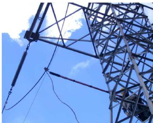
Figura 42: Aterrando as fases.
